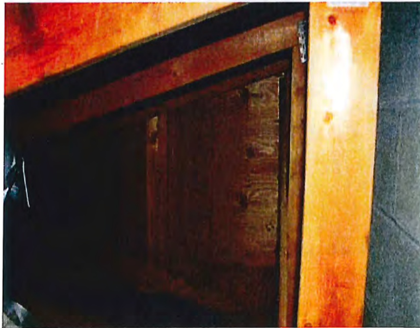
Figure F.4 Plywood sheathing at gable end wall
