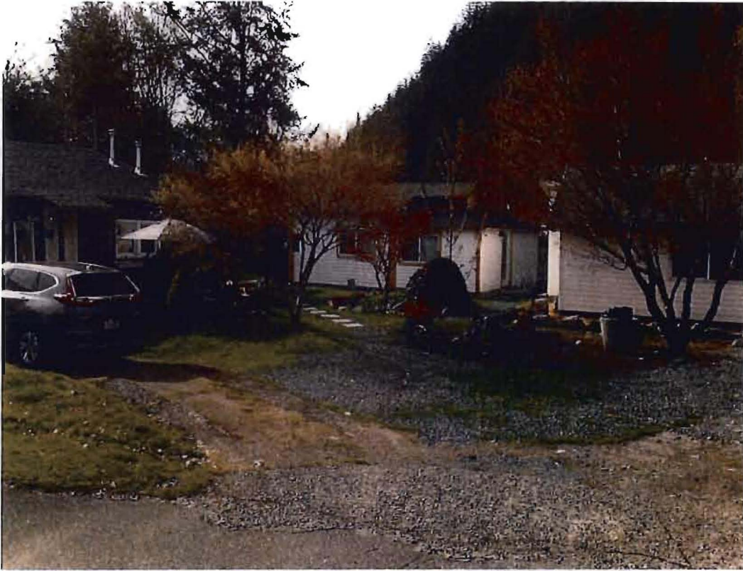
Photograph 3. Typical view of the subject property from Cedar Avenue, facing south. This area is entirely within the SPEA.
