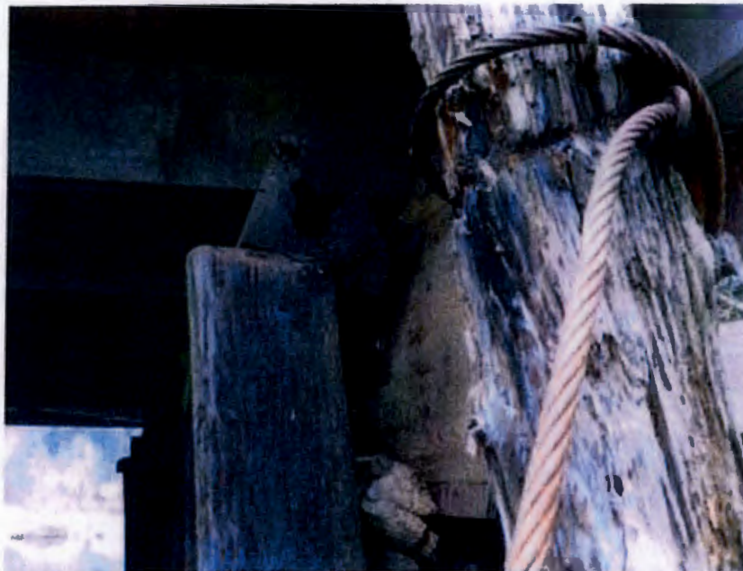
Photo 7: Cap beam and timber pile connection at north abutment. Note severe decay of cap beam.
