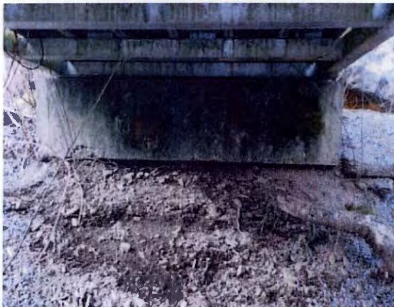
Photo 4: View of concrete abutment at west end. Light honeycombing at bottom left corner
