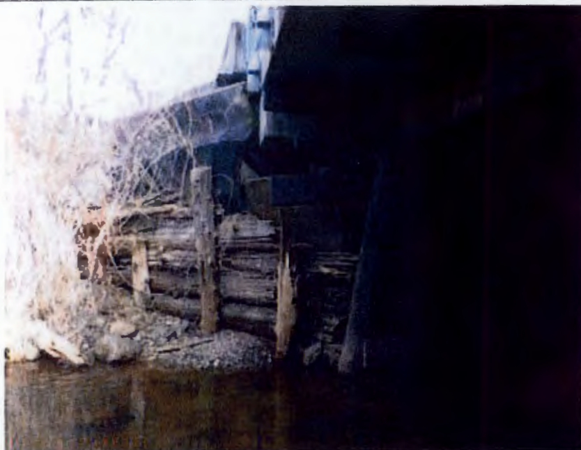
Photo 5: Timber piles and ballast logs at wingwall
