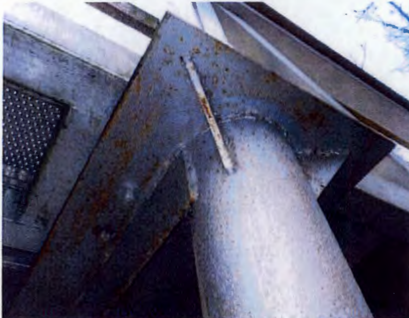
Photo 5: Minor general corrosion of protective coating at steel members
