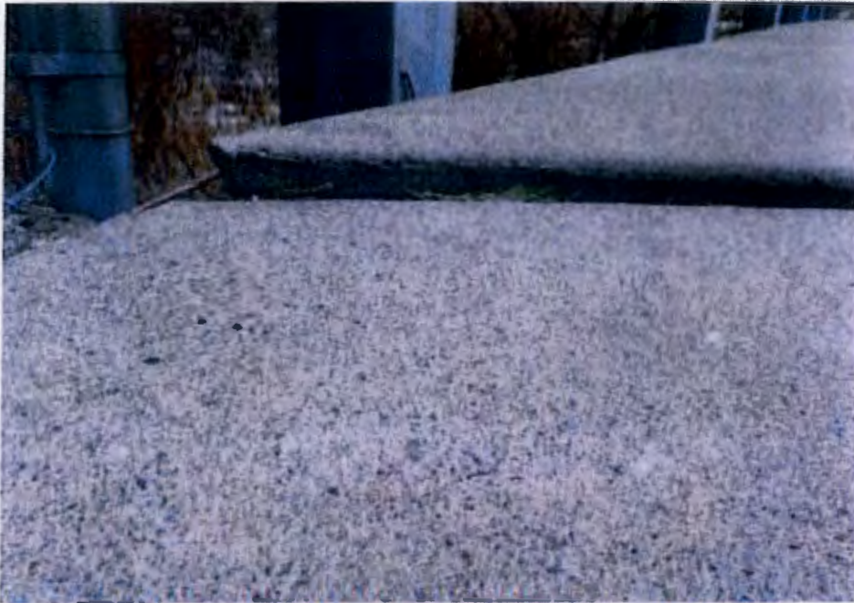
Photo 3: Differential settlement at sidewalk at bridge/approach interface
