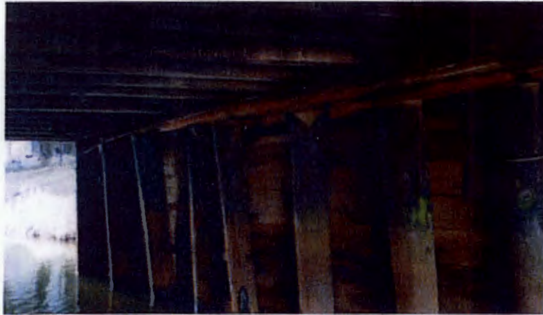
Photo 5: North abutment - note cap beam severely split and no longer bearing on top of piles
