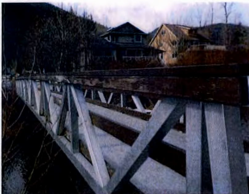
Photo 6: Side view of bridge. Full coating of paint was only applied on the inside face of the bridge.
