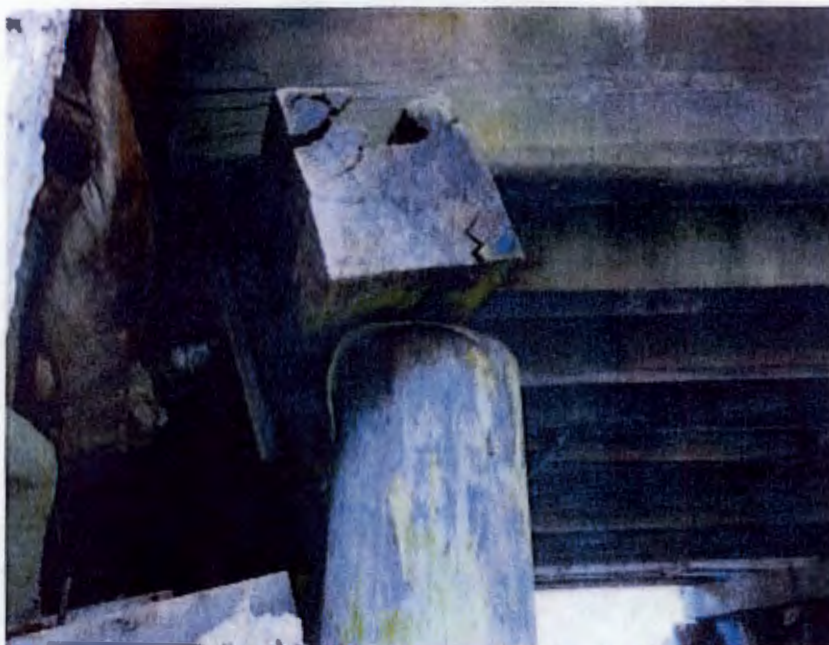
Photo 6: Cap beam and timber pile connection at south abutment
