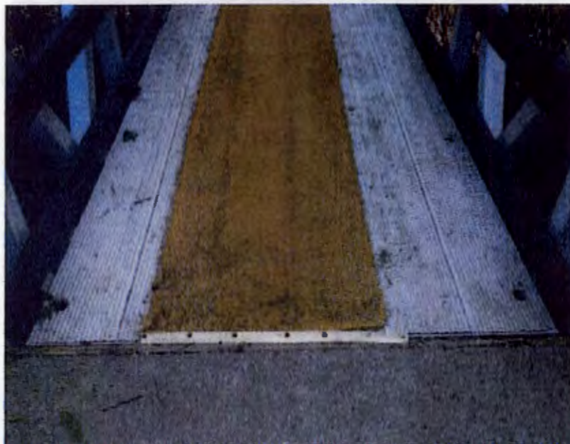
Photo 6: Caps missing at deck channels. Traction mat starting to loosen from support.
