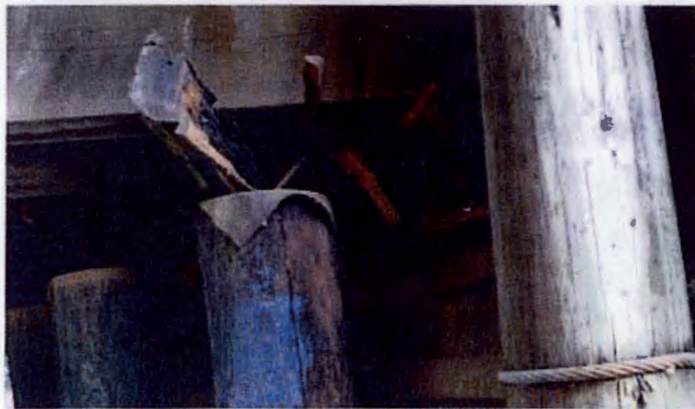
Photo 6: South abutment - note cap beam severely split and large gap between pile and ballast boards
