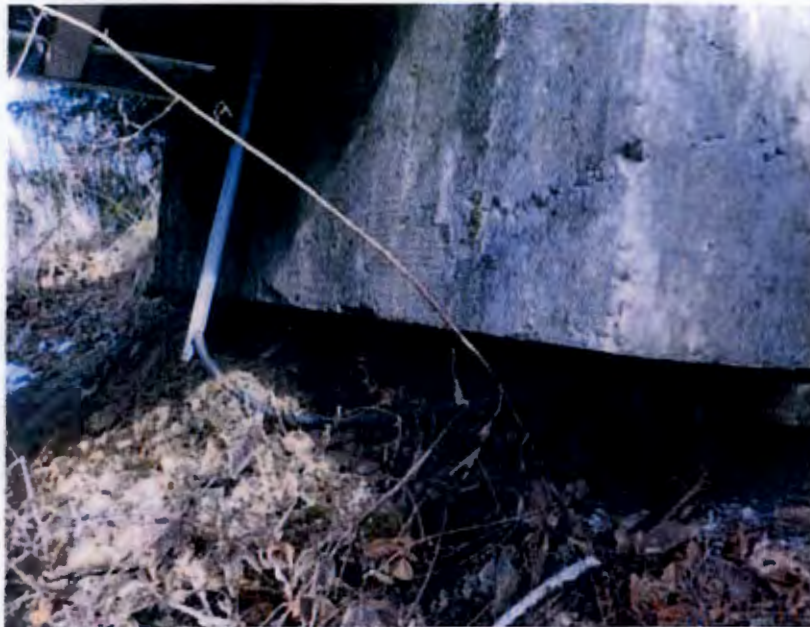
Photo 5: View of concrete abutment at east end. Erosion of abutment should be monitored.
