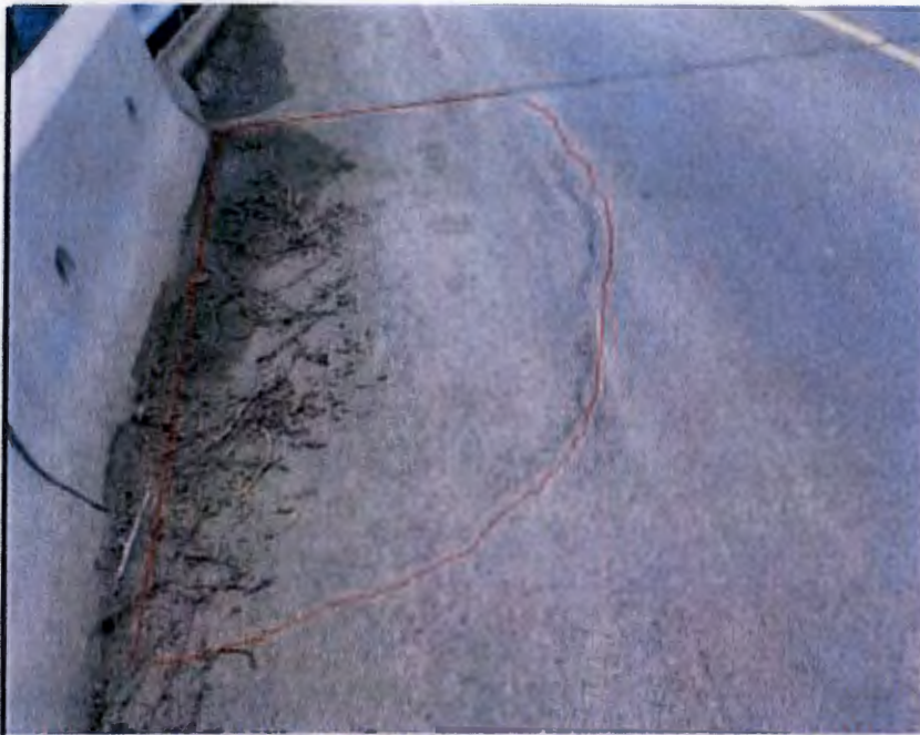
Photo 3: Localized settlement visible between asphalt crack and road barrier
