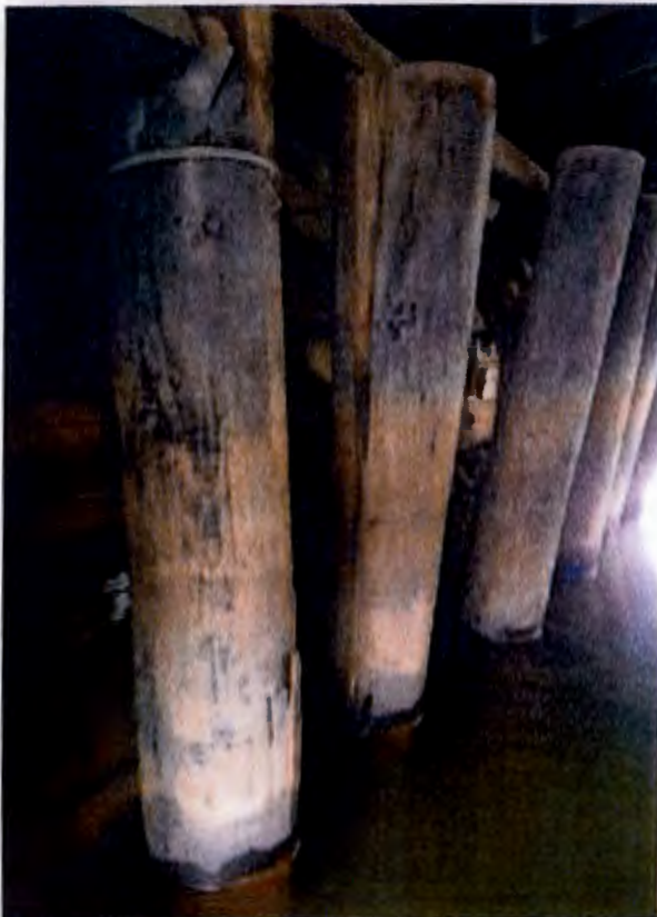
Photo 4: South abutment – Left pile cracked near bottom. Adjacent pile has severe split.
