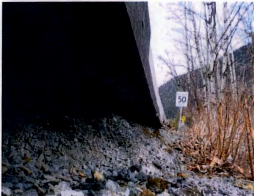
Photo 4: View of underside of road barrier showing extent of bearing material erosion
