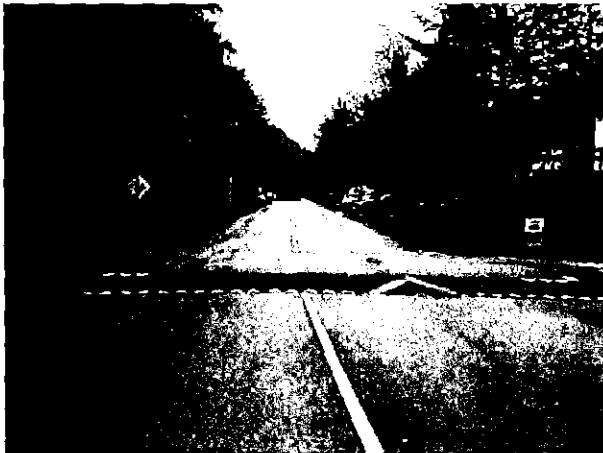
Figure 3.3: Example of a Raised Intersection
