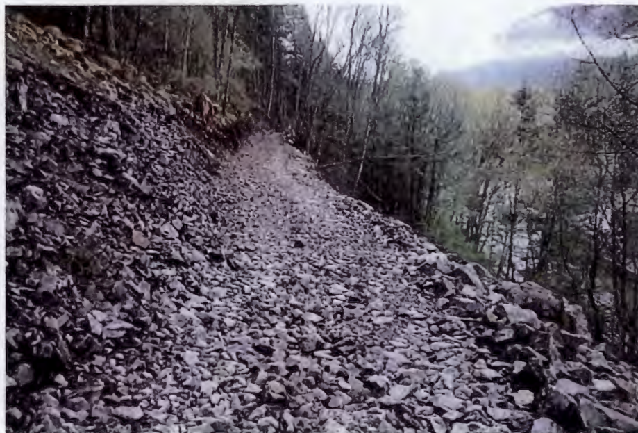
Photo 4. Looking south from HL5 at the constructed road.
