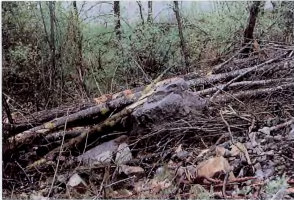
Photo 3. Looking west from HL7 at the hillslope. Medium to large size boulders held up by timber poses significant hazard to public road down below; required to be hauled up/retrieved.
