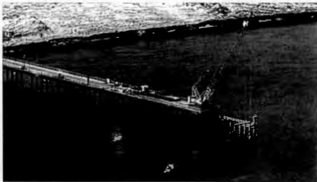
The 329-metre Peace River construction bridge was completed in March 2016, linking the north and south banks of the dam site.
