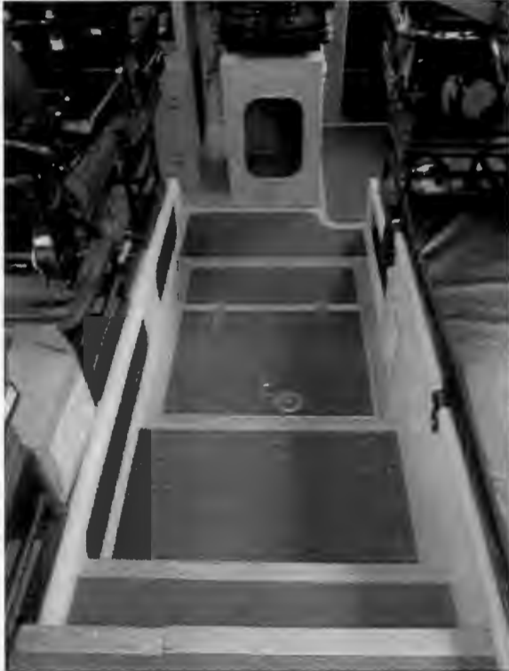
Renovate cabin flooring and deck surfaces
