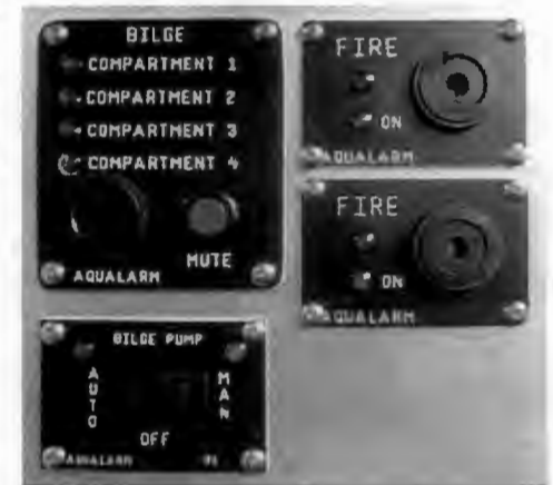
Install bilge and fire alarms
