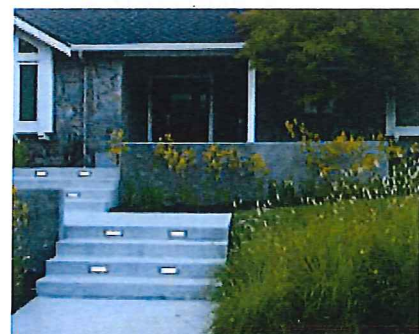
CONCRETE STAIRS W/ RECESSED STEP LIGHTS
