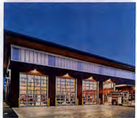
SILGA -- Southern Interior Local Government Association: Town of Osoyoos for the Osoyoos Fire Hall Courtesy: Wood Design Awards in BC
