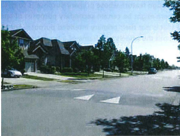
Figure 3.2: Example of a Speed Hump
