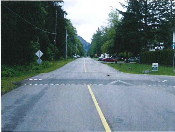
Figure 3.3: Example of a Raised Intersection
