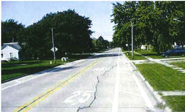
Figure 3.7: Example of Narrow Lane Markings
