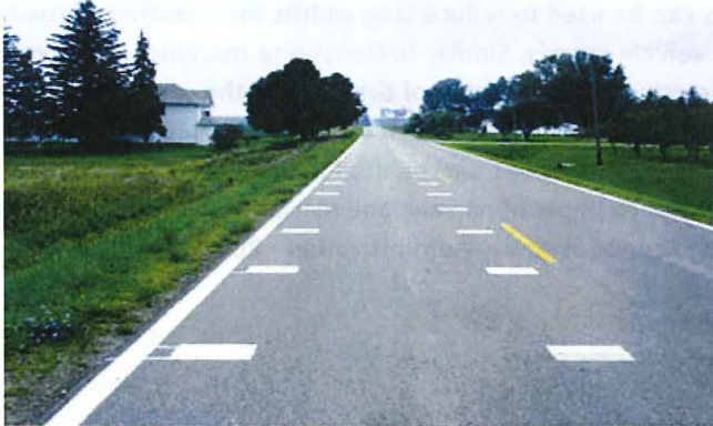
Figure 3.5: Example of Transverse Markings
