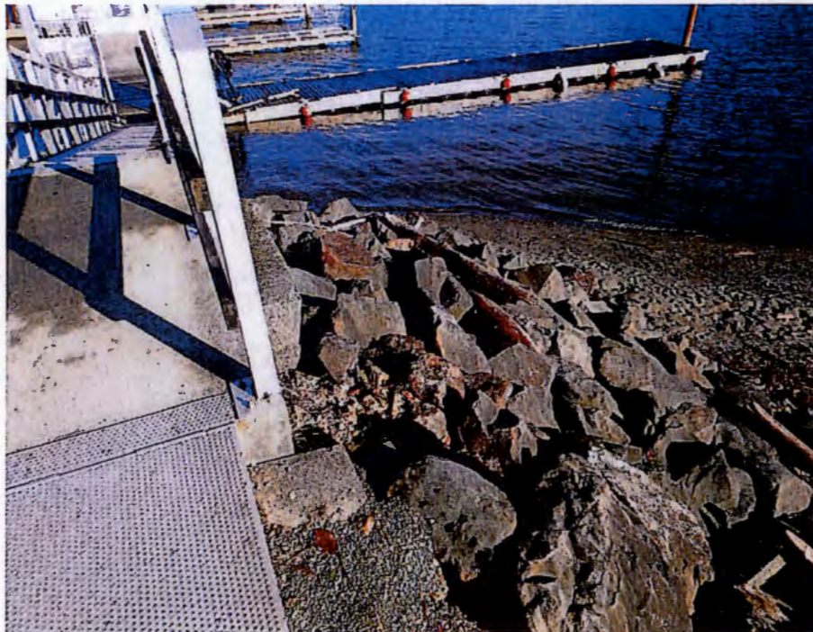
Figure 3.12 Zone 4 – Riprap protecting marina gangway abutment.
