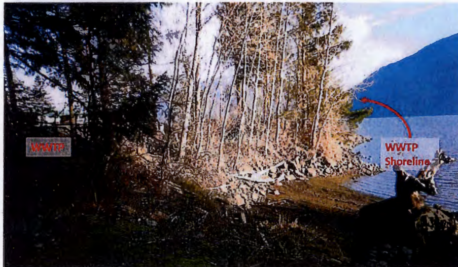
Figure 3.3 Zone 1 – View of the WWTP shoreline from the south.
