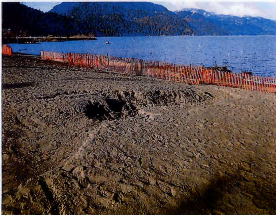
Figure 3.23 Zone 6 – Scour occurring at the top of the beach.
