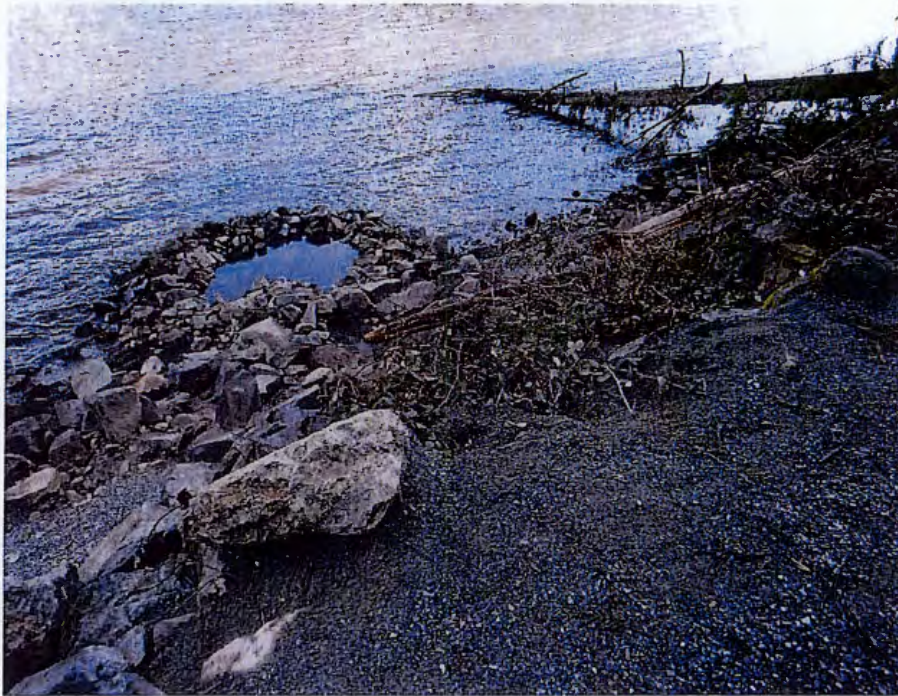
Figure 3.7 Zone 2 – Rock from the riprap slope removed to create warm pools.
