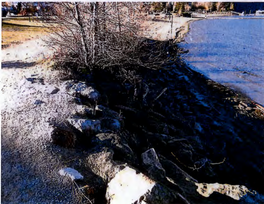
Figure 3.15 Zone 4 – Riprap slope at the transition to the Harrison lagoon.
