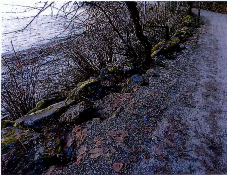
Figure 3.5 Zone 2 – Repaired erosion along the top of the riprap slope.
