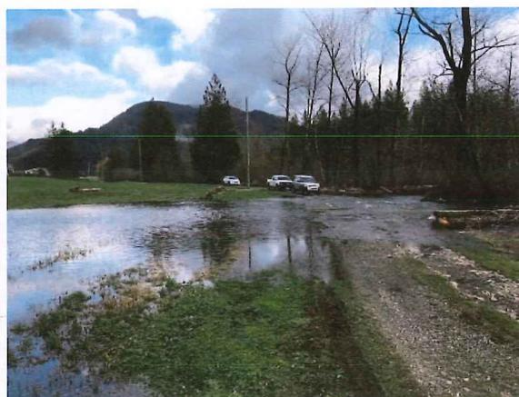
**Figure 3-4: Road washout caused by landslide redirecting flows from Hicks Creek. Site 02D.**
