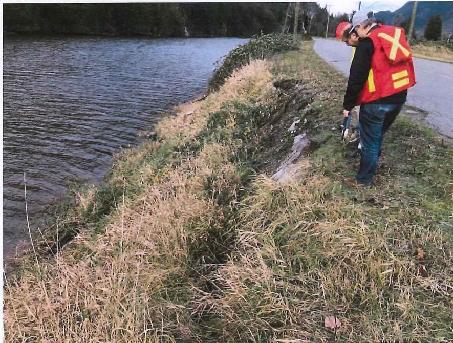
Figure A-2: Tetra Tech staff measuring sloughing section along Seabird Island Road
