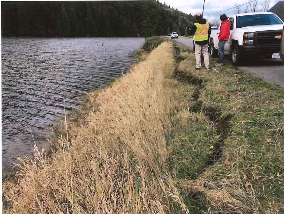
Figure A-1: Section of Seabird Island Road embankment sloughing - approximately 50 m long
