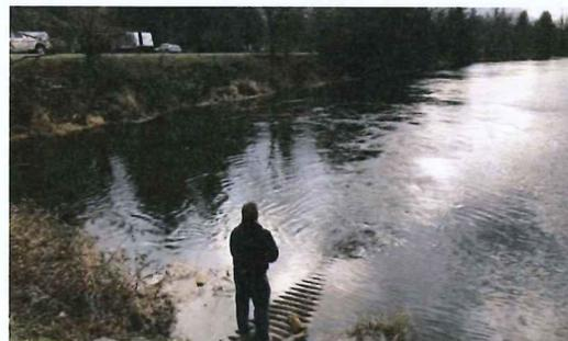
Figure 3-12: Surcharged culvert servicing private driveway
