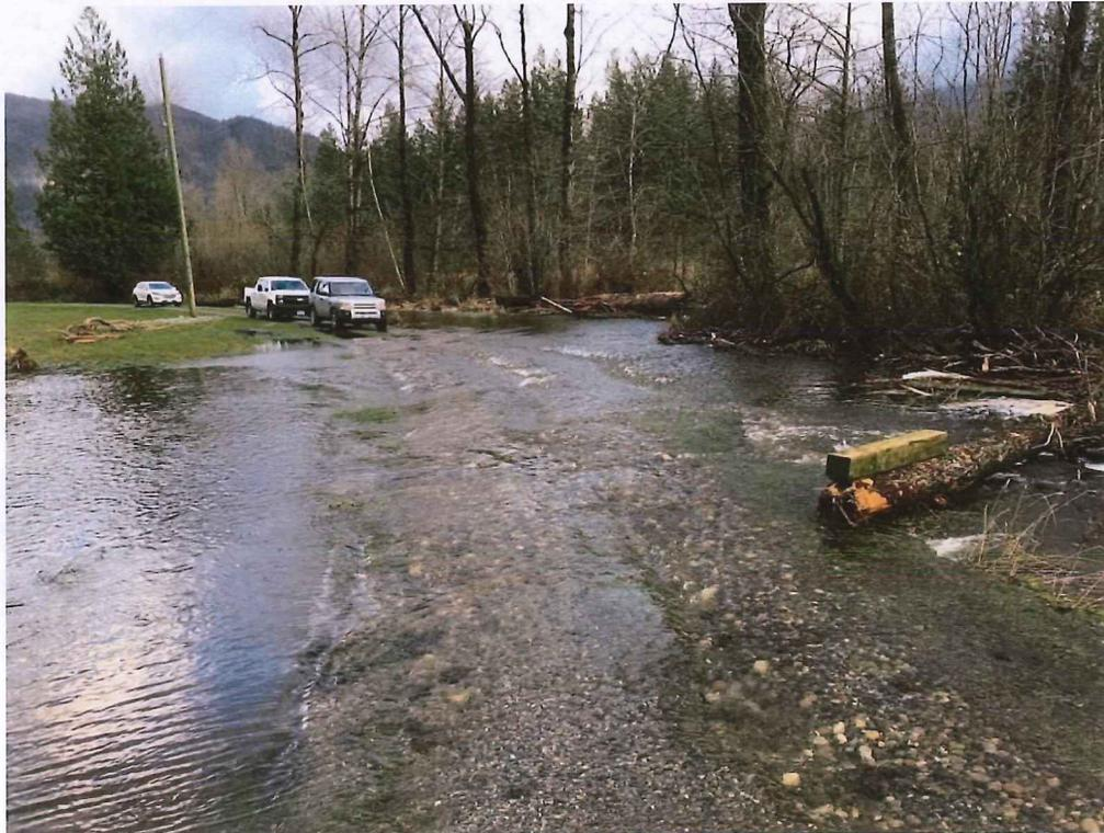
Figure A-10: Road washout due to channel blockage. Site 02D
