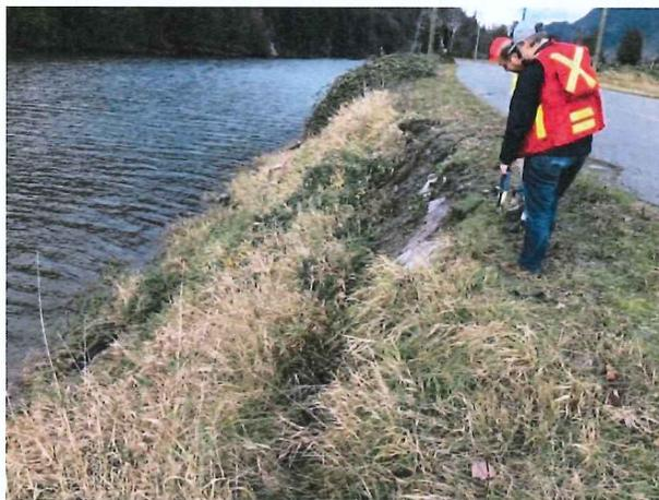
Figure 3-1: Tetra Tech staff measuring sloughing on the west side of Seabird Island Road
