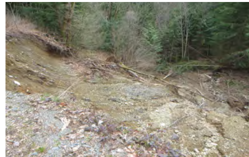
The old Harrison East FSR roadbed washout #1
