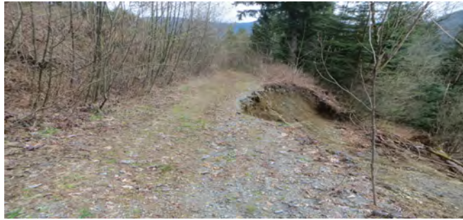
The old Harrison East FSR roadbed washout #1
