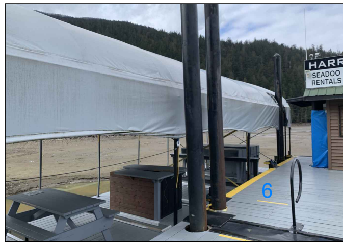
EPOXY COATED STEEL PIPE ANCHOR PILES
