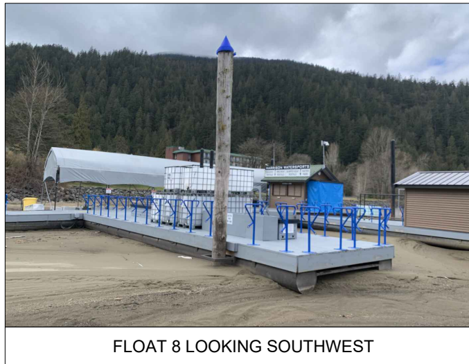
FLOAT 8 LOOKING SOUTHWEST
