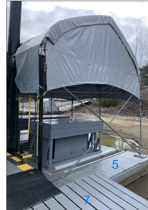
FLOATS 5 & 7 LOOKING SOUTHEAST
