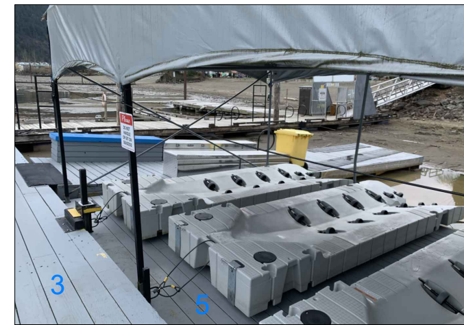
JET SKI LIFTS MOORAGE ON FLOAT 5
