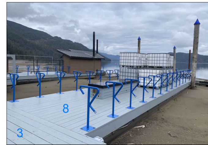
FLOATS 3 & 8 LOOKING NORTHWEST
