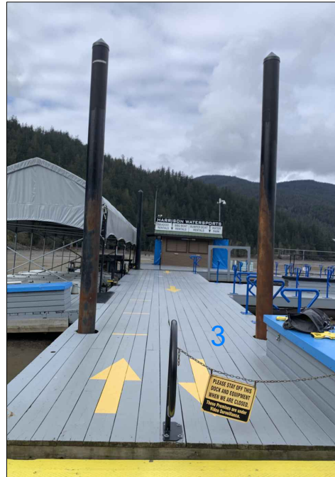
FLOAT 3 LOOKING WEST
