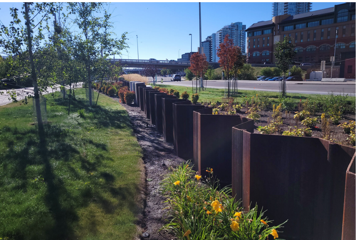
Sheet pile flood wall RiverWalk - Calgary, AB
