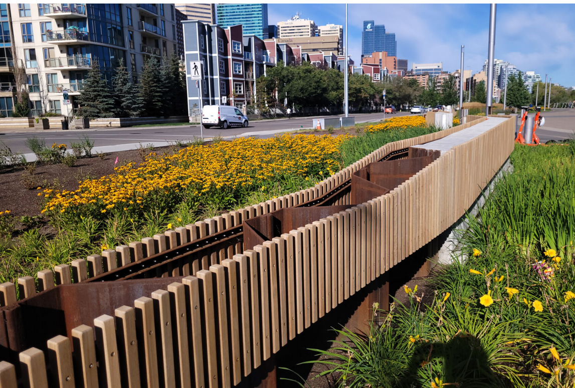
Sheet pile flood wall with custom cladding RiverWalk - Calgary, AB
