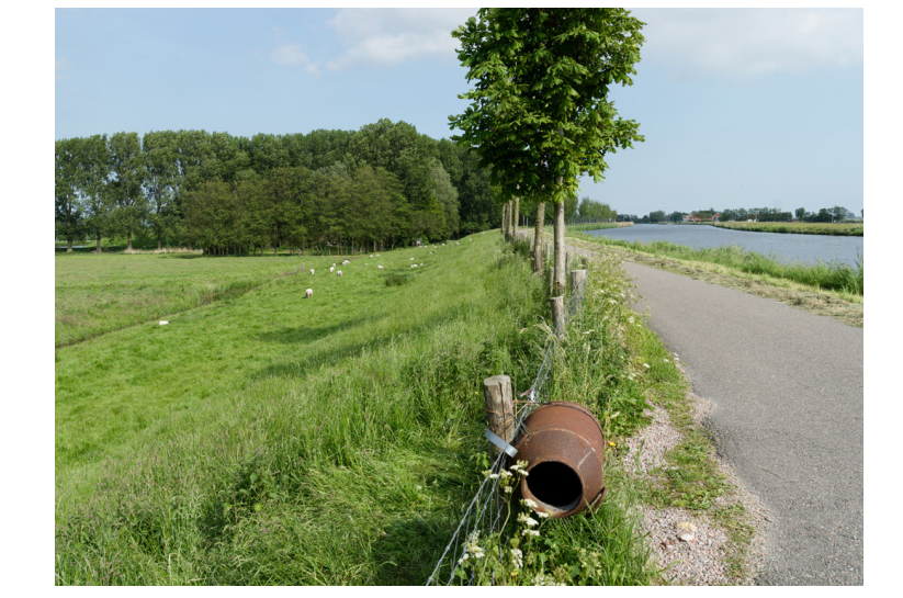
Earthfill dike as flood protection Netherlands
