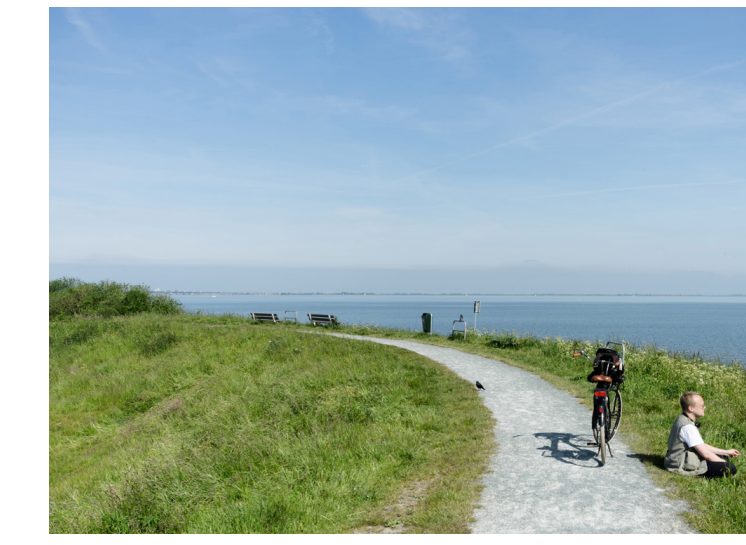
Earthfill dike as flood protection Netherlands
