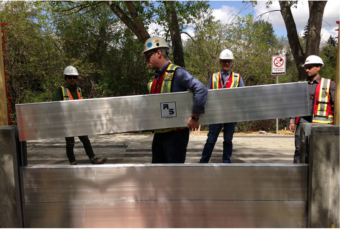
Installation of demountable aluminum flood barrier RiverWalk - Calgary, AB
