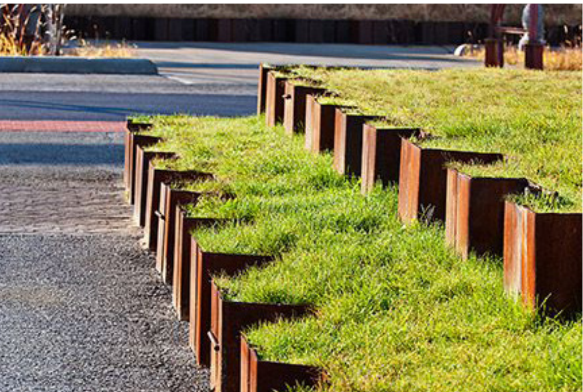
Two tiers of sheet pile walls The Steel Yard - Providence, RI
