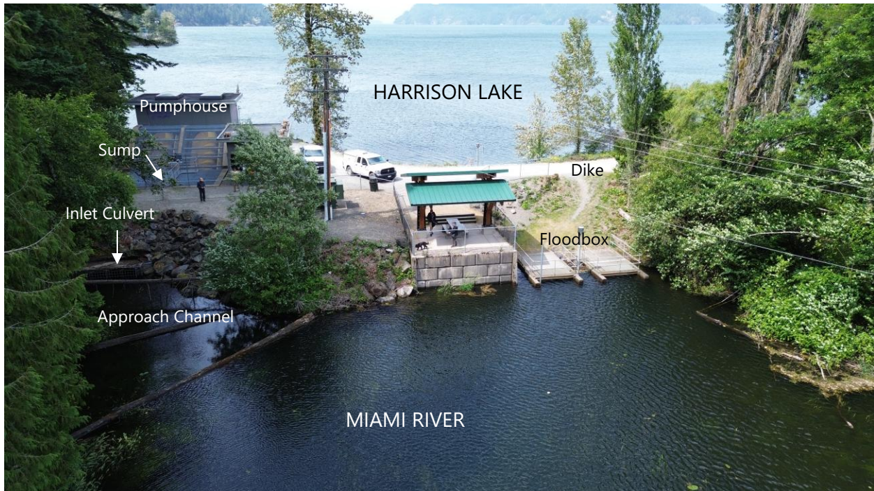
Figure 1.2 Miami River Pump Station, viewed from upstream (NHC photo, May 21, 2025)
