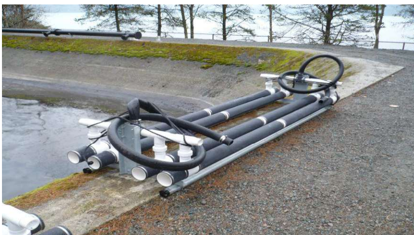
Figure 10. Bioreactor Aeration Diffuser (typ.)
