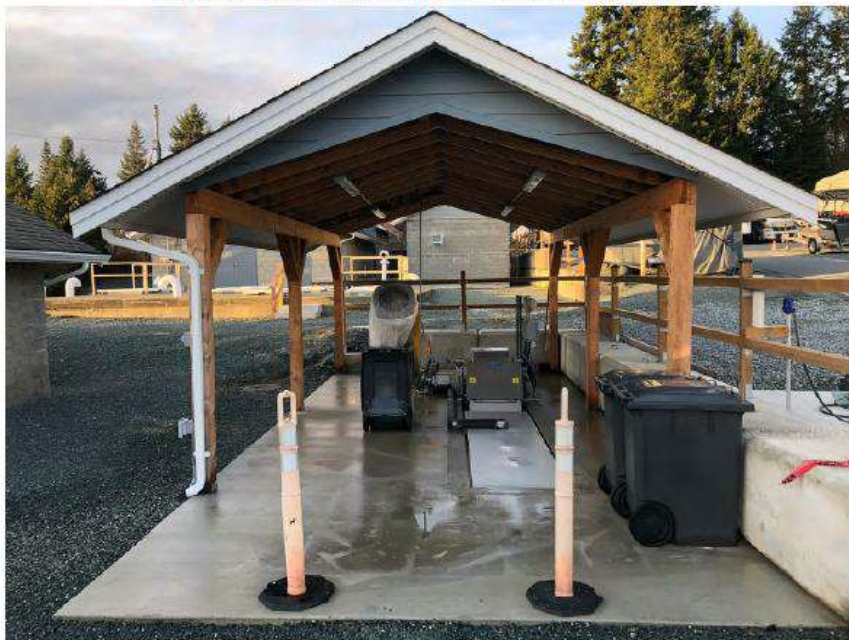
14. Arbutus Ridge WWTP, BC (Cowichan Regional Valley District, BC; March 2019; Preselected; Protection of MBR) – McElhanney Project
