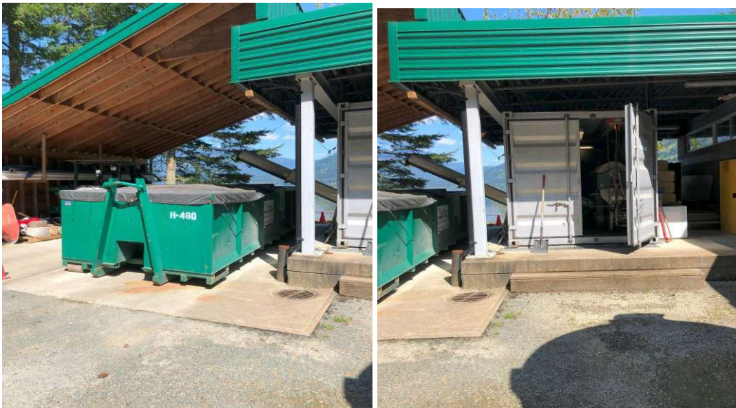
Figure 16. Centrifuge System. Roof cover over solids disposal bin (left); centrifuge in seacan (right).
