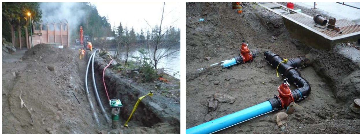
Figure 8. 2012 Forcemain Twinning from Miami River Pump Station to WWTP. a) Twinning along the pathway to the WWTP. b) Connection of twinned lines at the WWTP before the influent fine screen channel.
