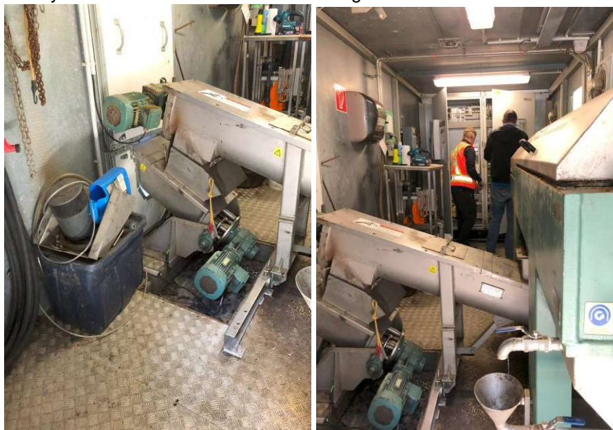
Figure 17. Centrifuge System. Two cake conveyors (left); limited maintenance room around the centrifuge (right).
