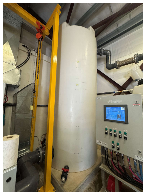
Figure 18: Break Tank
