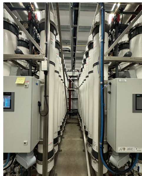
Figure 14: Ultrafiltration Membranes, Two Trains
