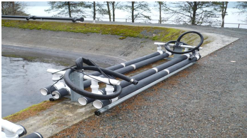
Figure 10. Bioreactor Aeration Diffuser (typ.)
