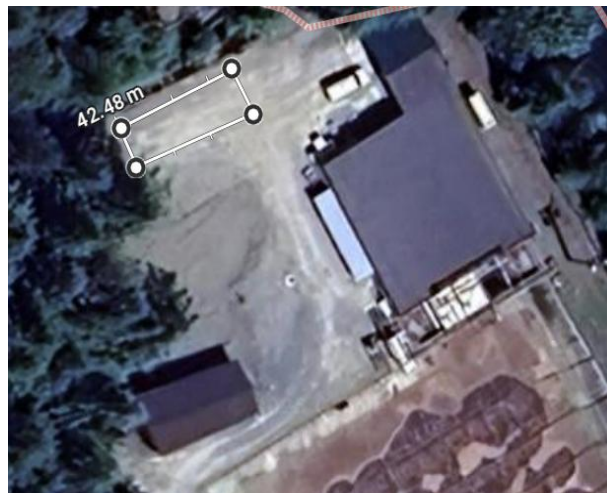
Figure 28. Approximate Area of 80 m 2 Operations Building in Northwest Corner of the Site
