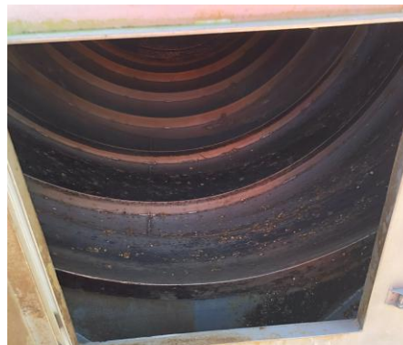
Figure 14. Inside of 2mm Drum Screen. Grit particles observable.
